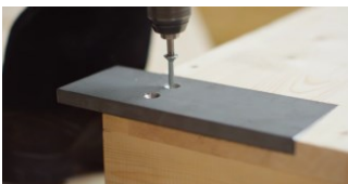
Large framing with trimmer and steel plates
