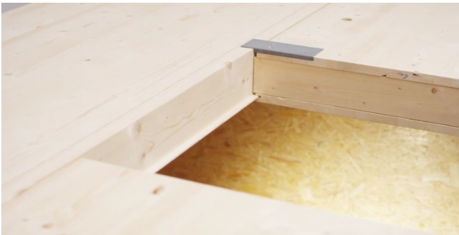
Large framing with trimmer and steel plates
